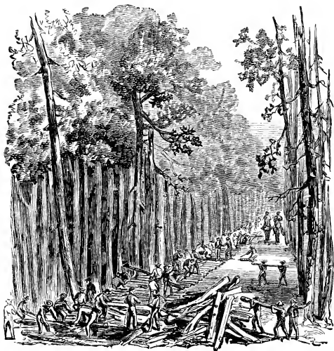
MAKING ROADS THROUGH NORTH CAROLINA.
